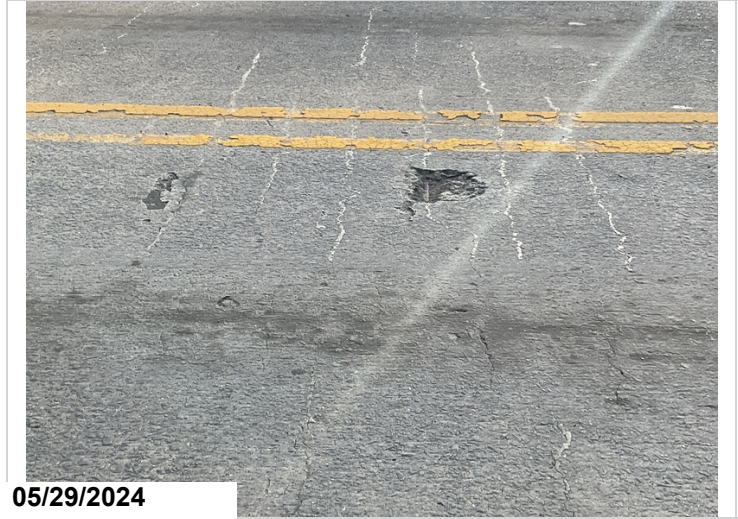
Span 1 at bent 1 southbound lane has a 1'x1' spall with rebar
