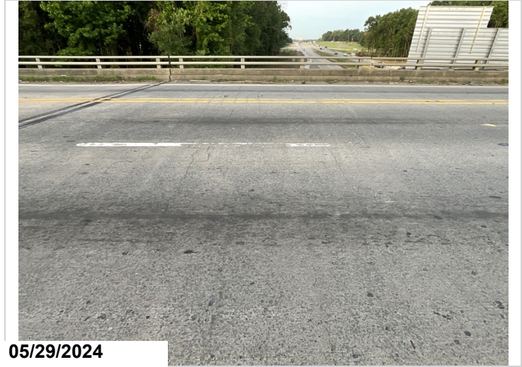
Sealed deck cracks in span 1.
