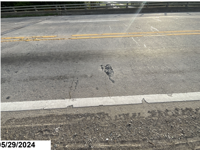
Span 2 at bent 3 1'x1' spall
