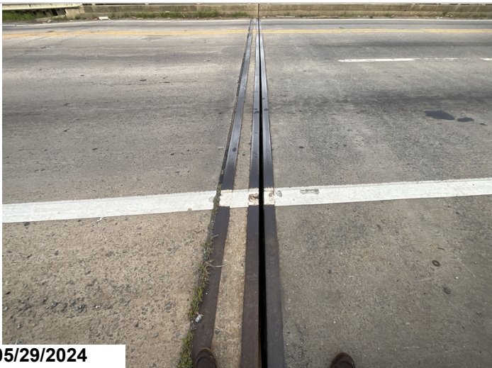
Bent 1 joint seal is missing
