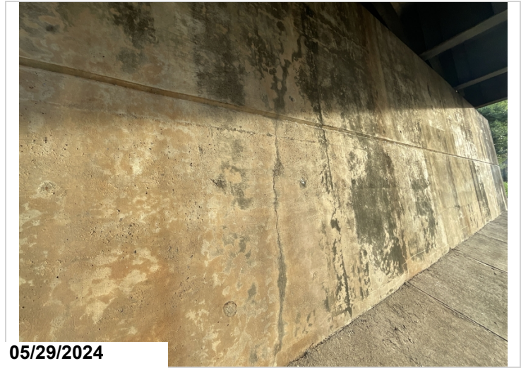
Vertical cracks in both abutments cs2
