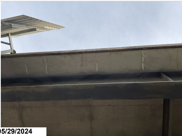
Efflorescence in the overhang
