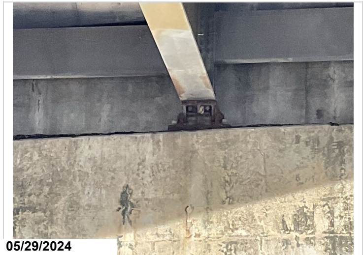
Bent 3 bearing 4 cs3 typical most bearings
