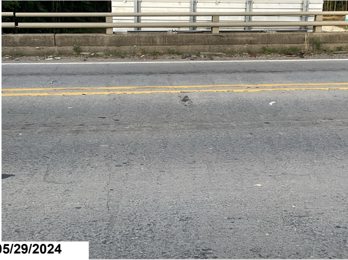
Span 1 middle lane has a 1'x1' spall cs2
