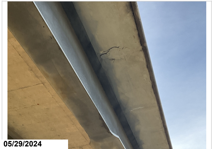
Span 2 at bent 3 left side has a 1'x1' delamination over slope pavement
