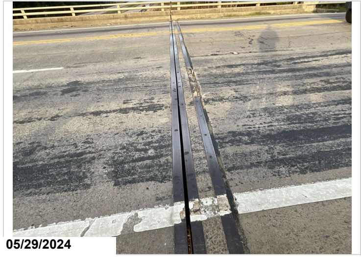
5' of armor is missing at bent 2 top of backwall
