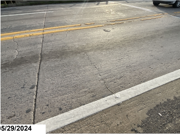
Bent 3 approach slab sealed transverse cracks
